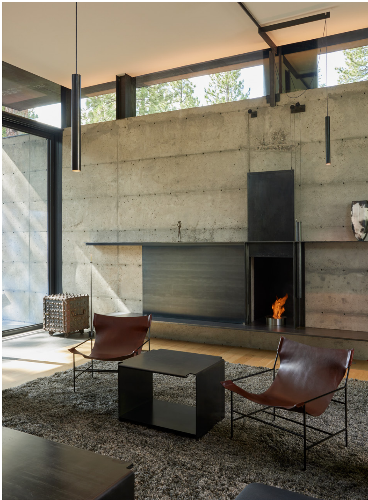
The double concrete walls and horizontal roofs insulate the interior and offer protection from the elements.
