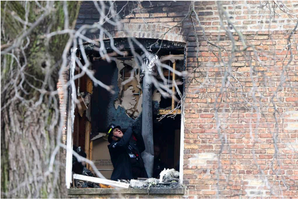
An official investigates an apartment building in the 500 block of West Marquette Road in Chicago's Englewood neighborhood where a 5-year-old girl died during a fire on Dec. 26, 2023. (Eileen T. Meslar/Chicago Tribune)
