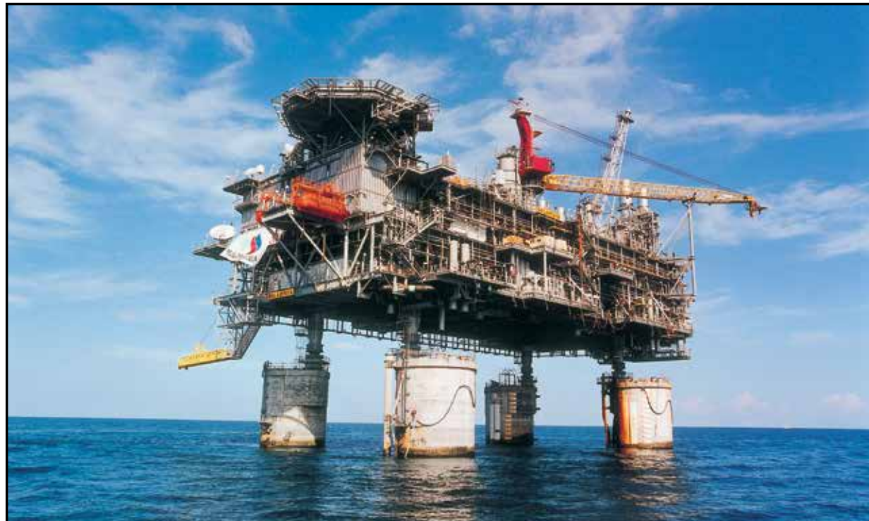
Emerson's automation upgrade enhances the reliability at the Malampaya natural gas production and processing facilities run by Shell Philippines Exploration B.V. (Photo courtesy of Emerson Automation Solutions)
