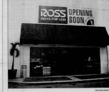
Ross Dress for Less, a discount clothing and home accessory store, will open a new shop at the Overseas Market in July. The storefront was left empty last summer by J.C. Penney because of declining sales. The department store, which laid off 50 employees, had been one of the few department stores in the Keys.
