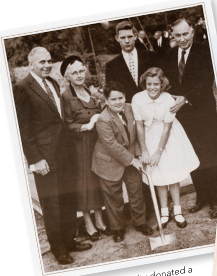
In 1956, Emory University donated a five-acre plot of land on its campus to construct a new Egleston Hospital with 100 beds.
