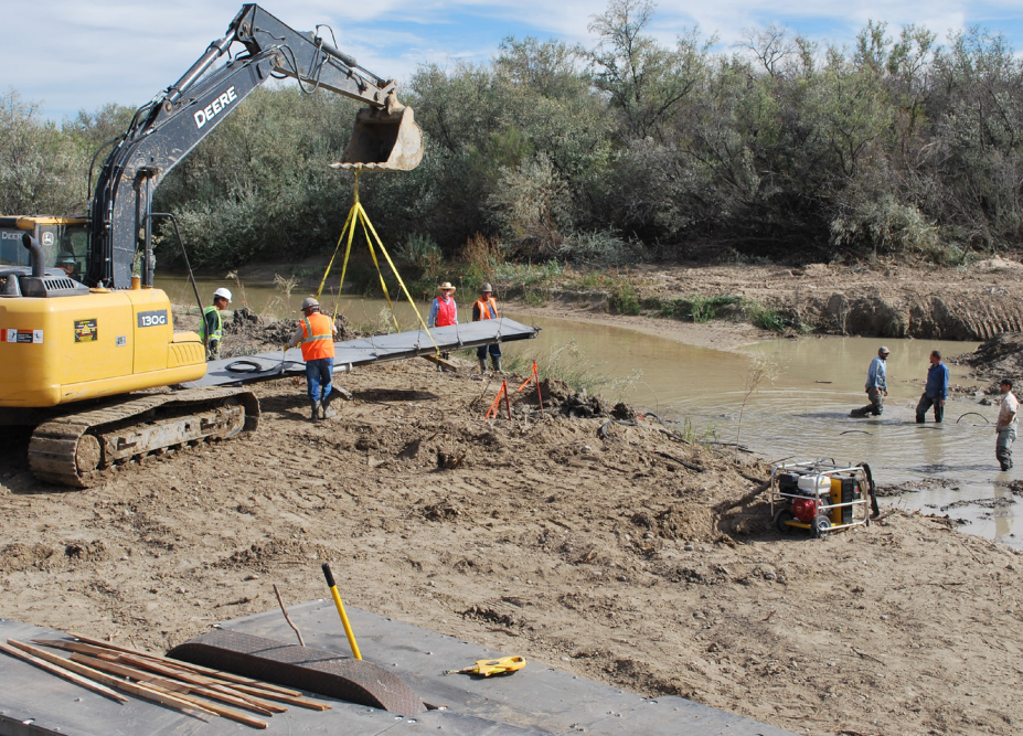
Installation of a flat-plate, pass-by antenna to track tagged fish in a shallow channel of the San Juan River. © Mark McKinstry
