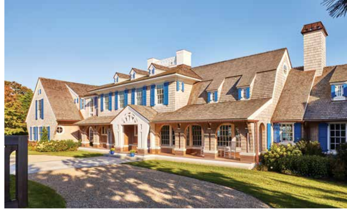
RIGHT: The center section of the twenty-year-old house was razed and rebuilt atop its old foundation in a mix of Federal and Dutch Colonial styles that suggest additions made over time. BELOW: The main staircase passes in front of an arcade of flattened Greek Revival columns dividing the entry hall from the family room. FACING PAGE: In the old kitchen, an appliance wall blocked the ocean view; now a custom lantern illuminates a Shaws sink in the island, which enjoys unobstructed ocean vistas.
