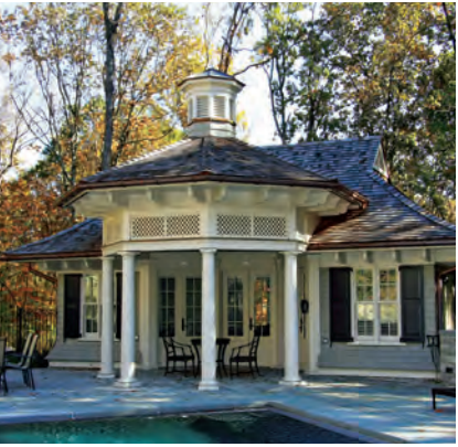
A Cornerstone-built pool house
