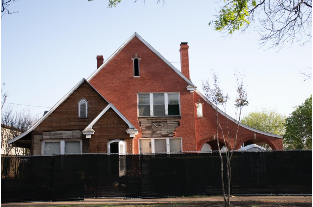
This 1920s Tudor-style home is one of the endearing structures set for demolition along Eighth Street. Local developer David Spence salvages the bricks, doors, and other historic features for his preservation/restoration projects in the area (England).
