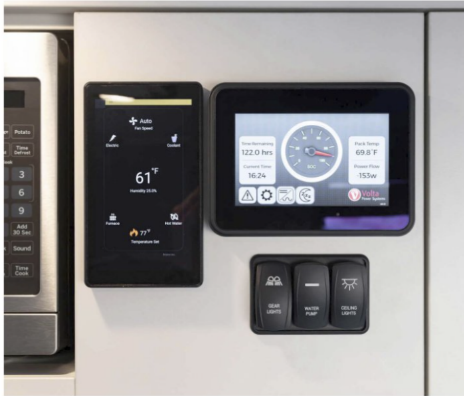
The control for Volta's 48-volt power system in the 2024 Outside Van Approach motorhome displays the batteries' state of charge, temperature and charge time remaining.
