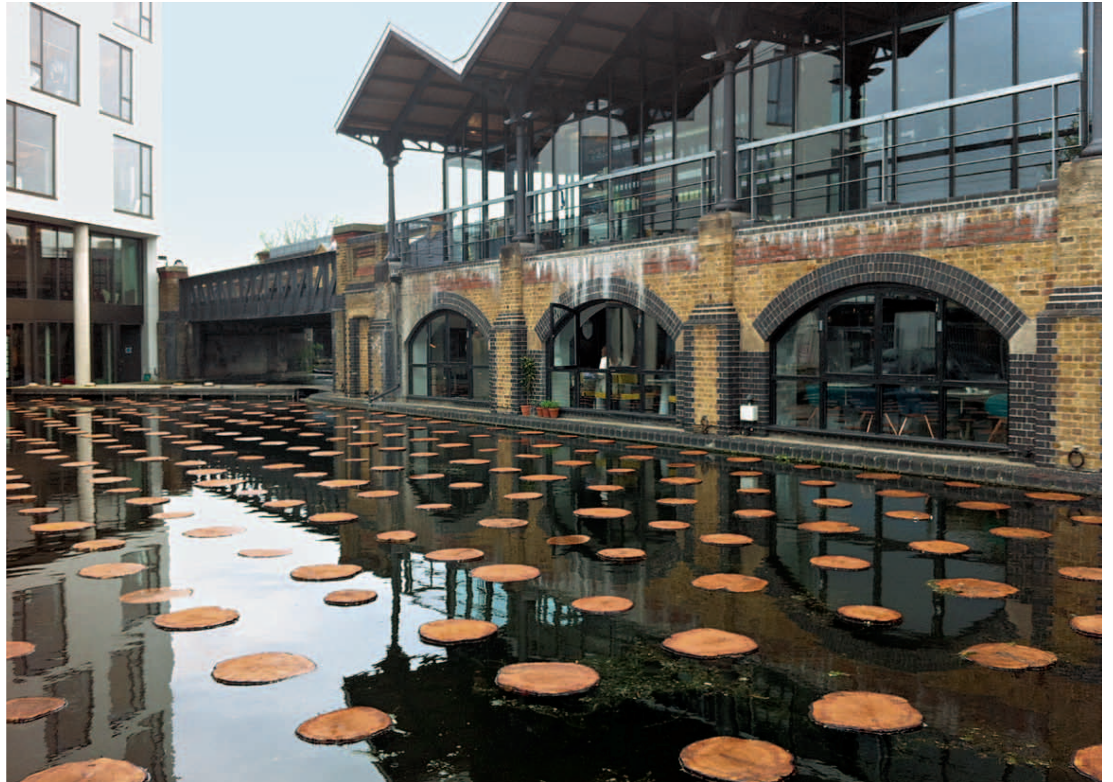
A grid of 450 floating timbers transform the Portobello Dock section of London's Grand Union Canal.
