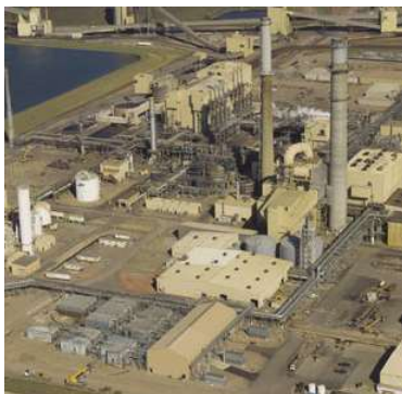
Coal Gasification Plant with CO 2 Capture
