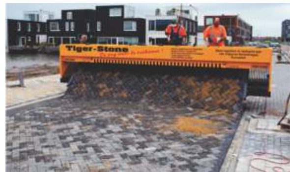
Brick Laying Through Robots (Source:- Egfi)
