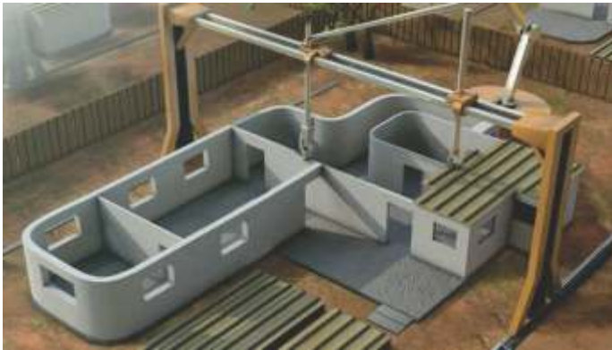
3D Printing A House (Source:- Giatech Scientific INC)
