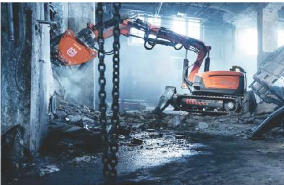
Demolition Works Through Robots (Source:-openPR.com)
