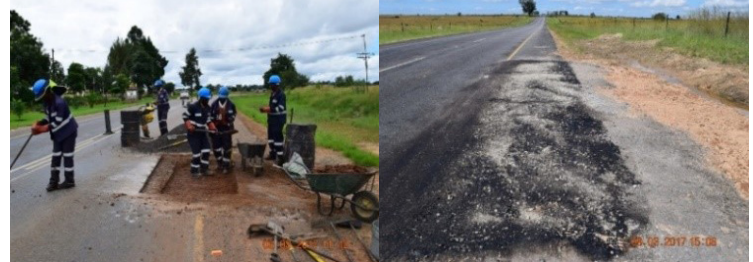
Figure 3: Edge repairs and completed repair of failed pavement
