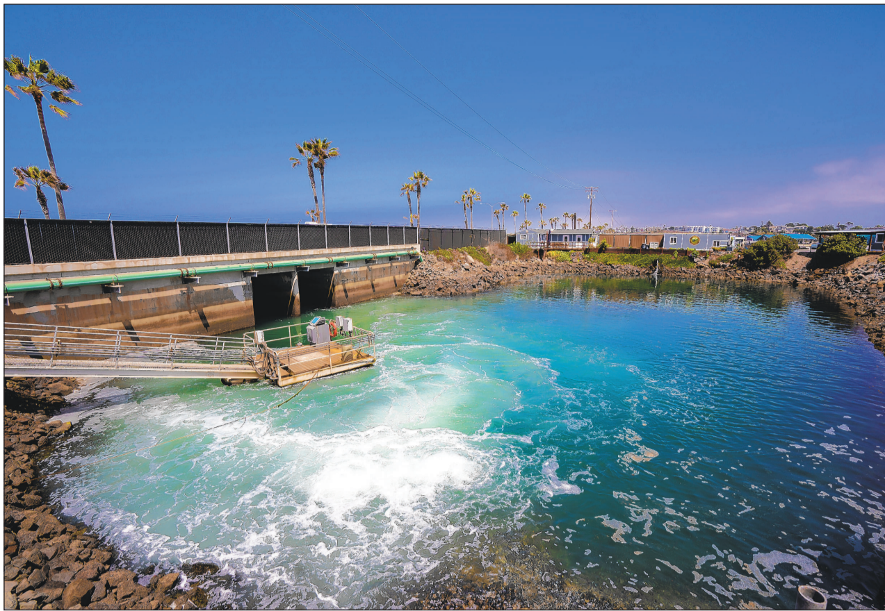
BRINE EXITING the Claude "Bud" Lewis Carlsbad Desalination Plant is further mixed with ocean water at the discharge pond. High concentrations of brine can raise toxicity in marine environments.
