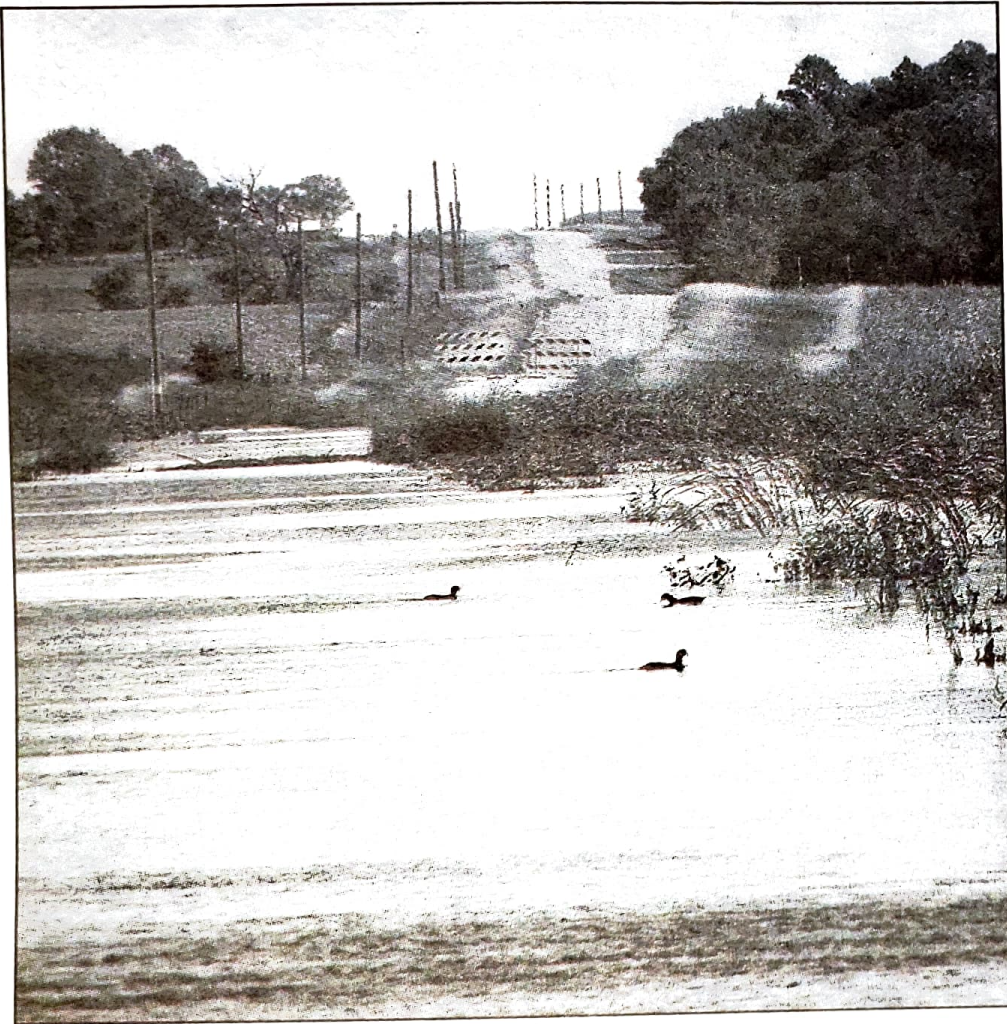
Culverts under the roads that cross over Lake Thompson's outlet cannot keep up with the rising water and 223rd Street has turned into a wetland where waterfowl swim peacefully across the road. (Times photo by Kerry Drager)
