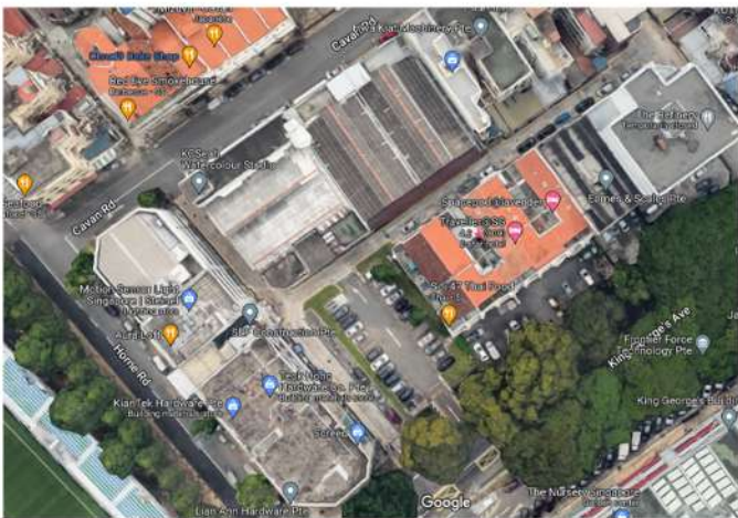
Proposed Site for Building Extension behind 7 Cavan Road, Carpark
