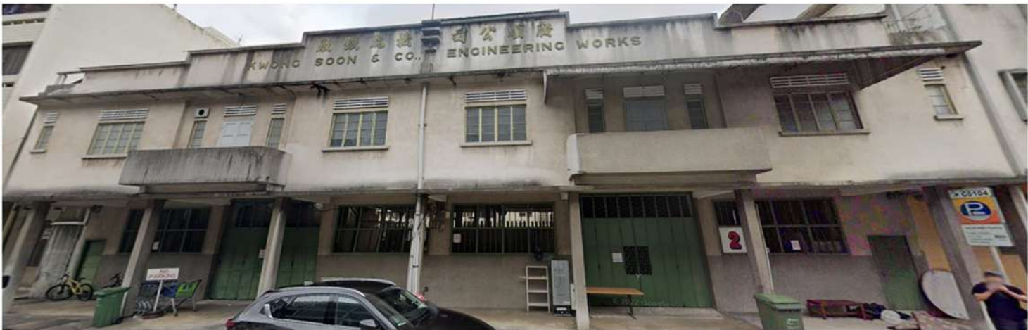
Exisiting Site Building Facade 2 Cavan Road
