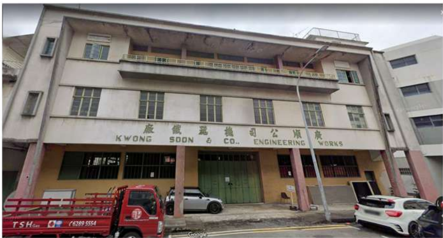
Exisiting Site Building Facade 7 Cavan Road
