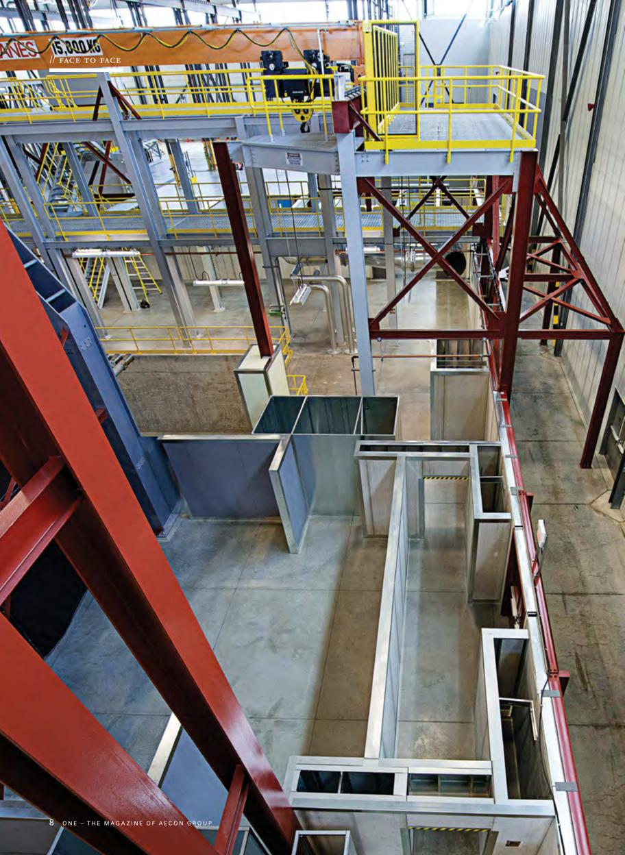
USING THE LATEST IN LASER SCANNING TECHNOLOGY, ALSO KNOWN AS OPTICAL METROLOGY, THE INSIDE OF THE UNIT 2 VAULT WAS SCANNED TO PRODUCE A MODEL THAT WOULD ASSURE ALL DIMENSIONS, INCLUDING STRUCTURAL STEEL AND WALL TOLERANCES, WERE AS ACCURATE AS POSSIBLE.
