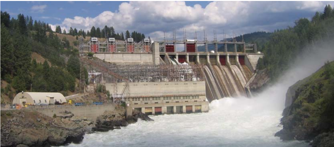
The Waneta Expansion Project is proposed to be built next to the current dam site in Trail (on the left in the above photo).
