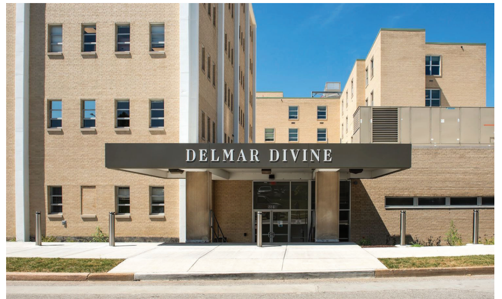
Built in the former St. Luke's Hospital, the Delmar DivINe is now an innovation hub serving nonprofits, with residential and company tenants.
