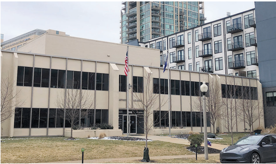
The Boy Scouts of America headquarters building.
