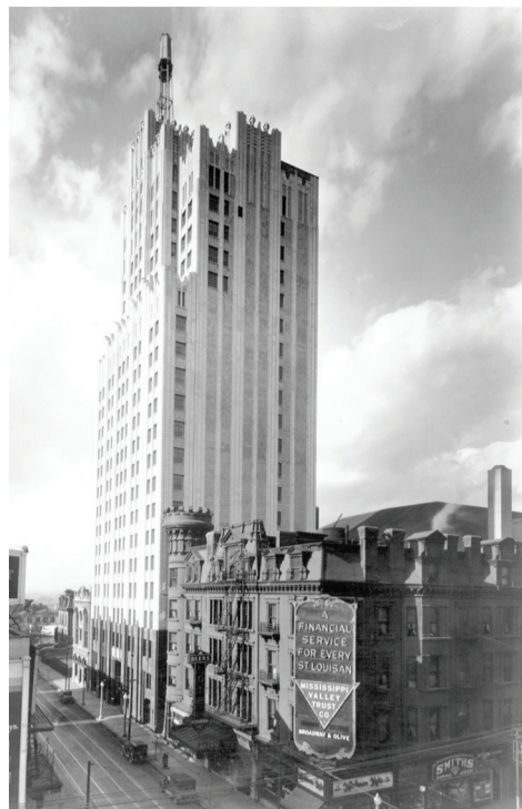
A historical photo of the Continental Building.
