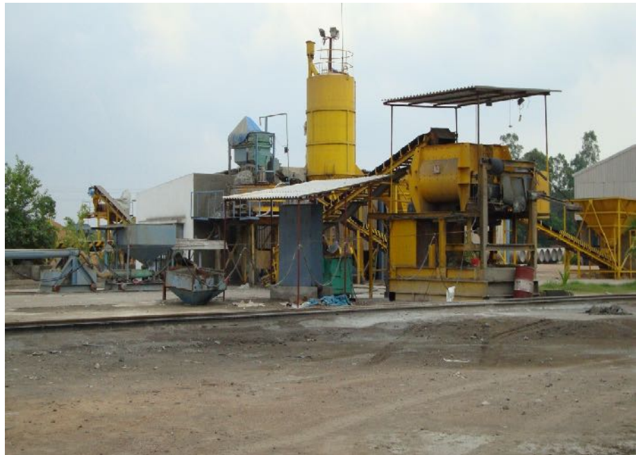
CML & Gunitting plant, Chennai
