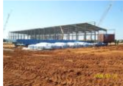
Formation building nearing completion.
