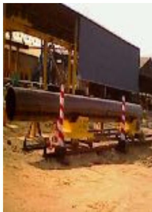
Pipe transfer and delivery to CML unit
