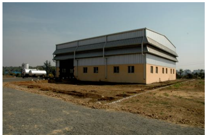
Biodiesel Plant – CCS, Daman
