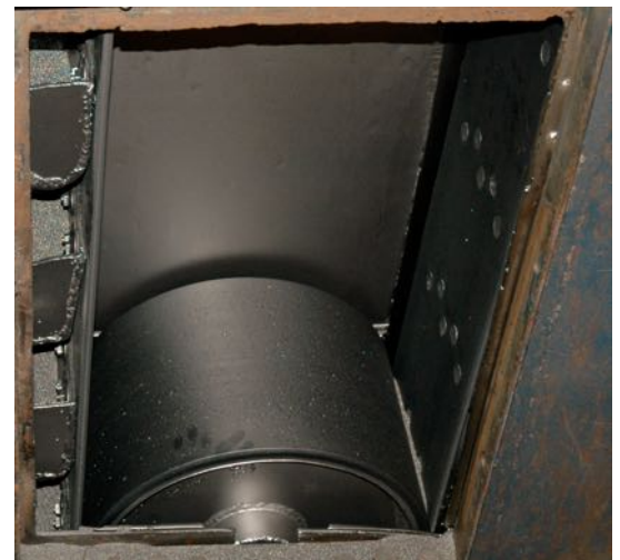
Rubber belt installed
