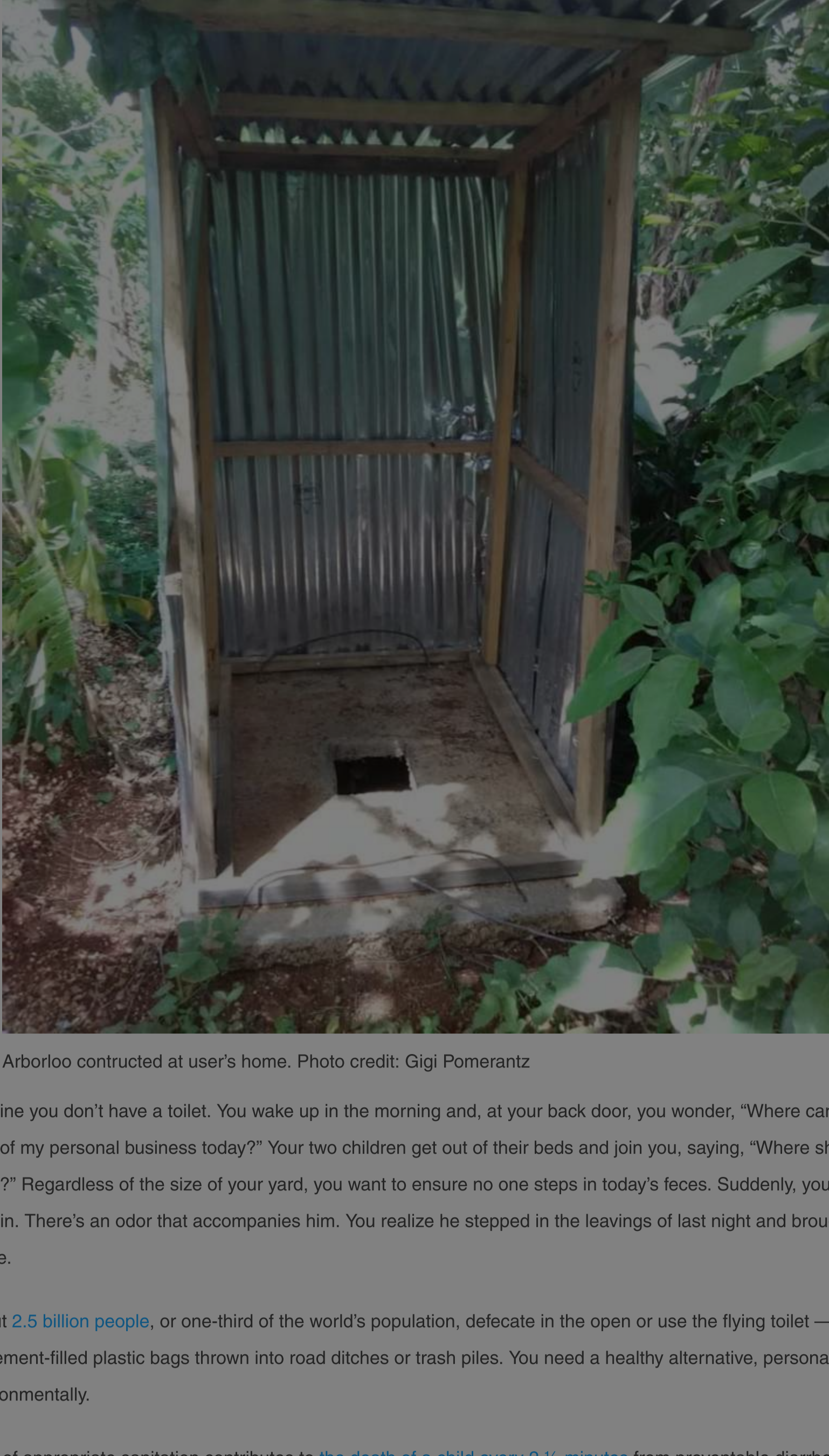
Arborloo constructed at user's home. Photo credit: Gigi Pomerantz
