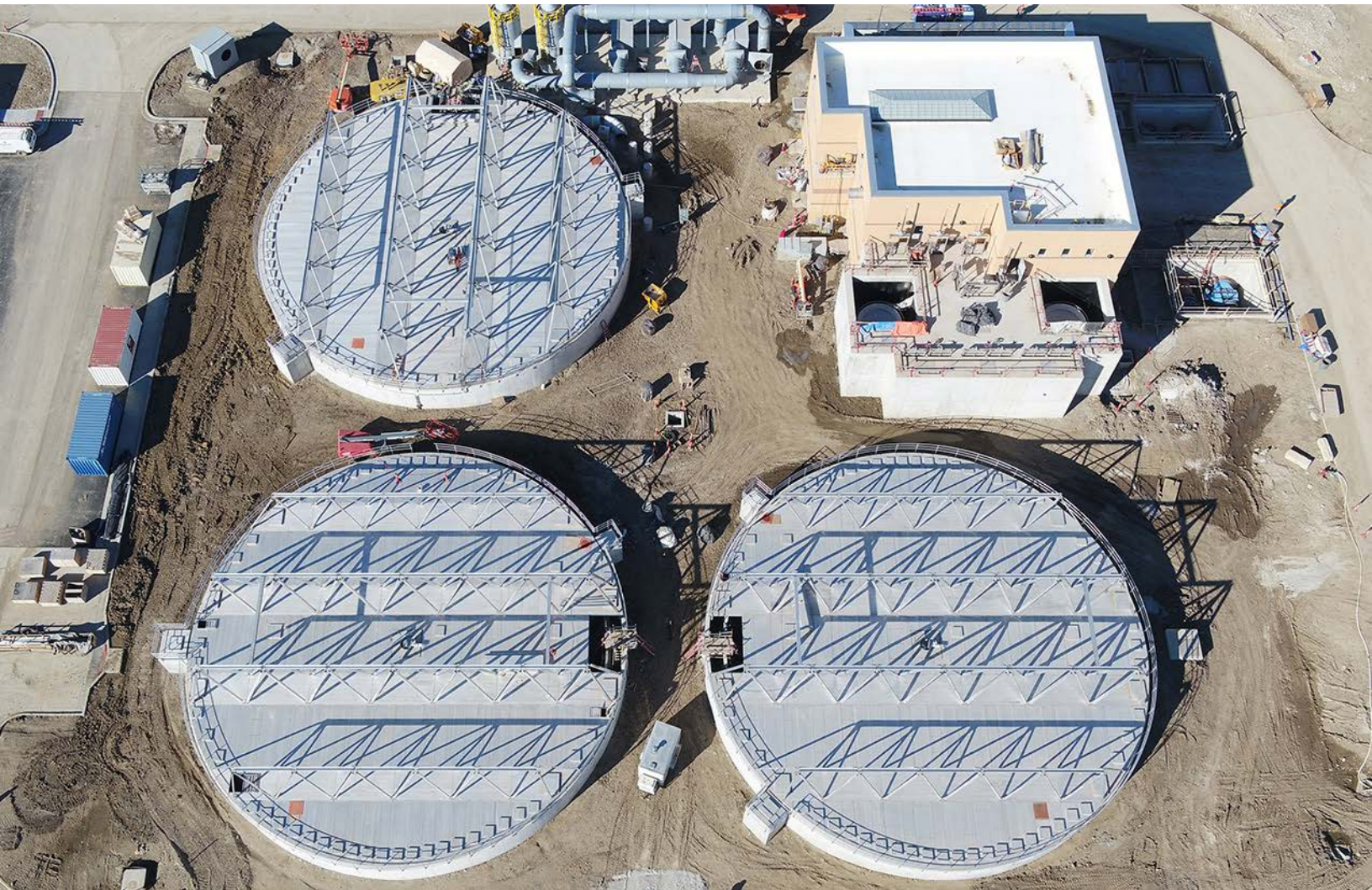
Headworks and primary clarifiers, March 1, 2021
