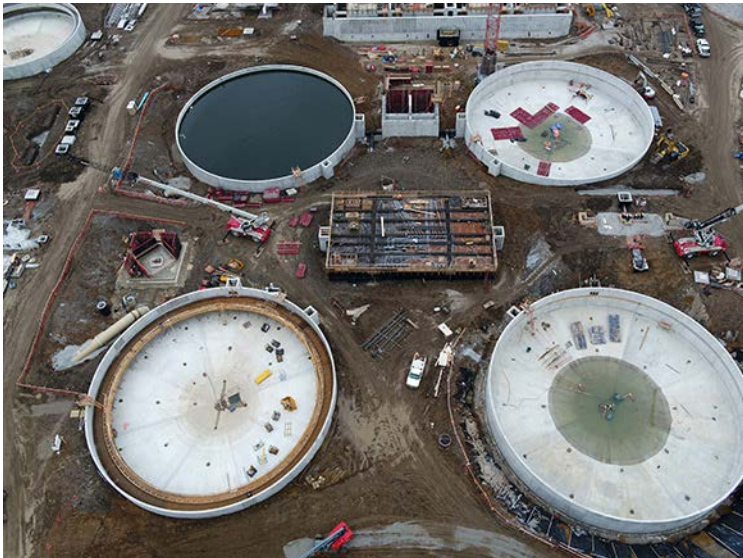
Final clarifiers, March 17, 2020
