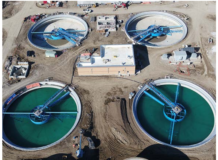
Final clarifiers, March 1, 2021
