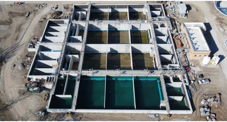
Overview of the BNR structure, March 1, 2021
