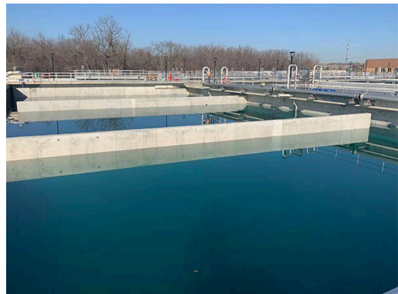
BNR structure, March 1, 2021
