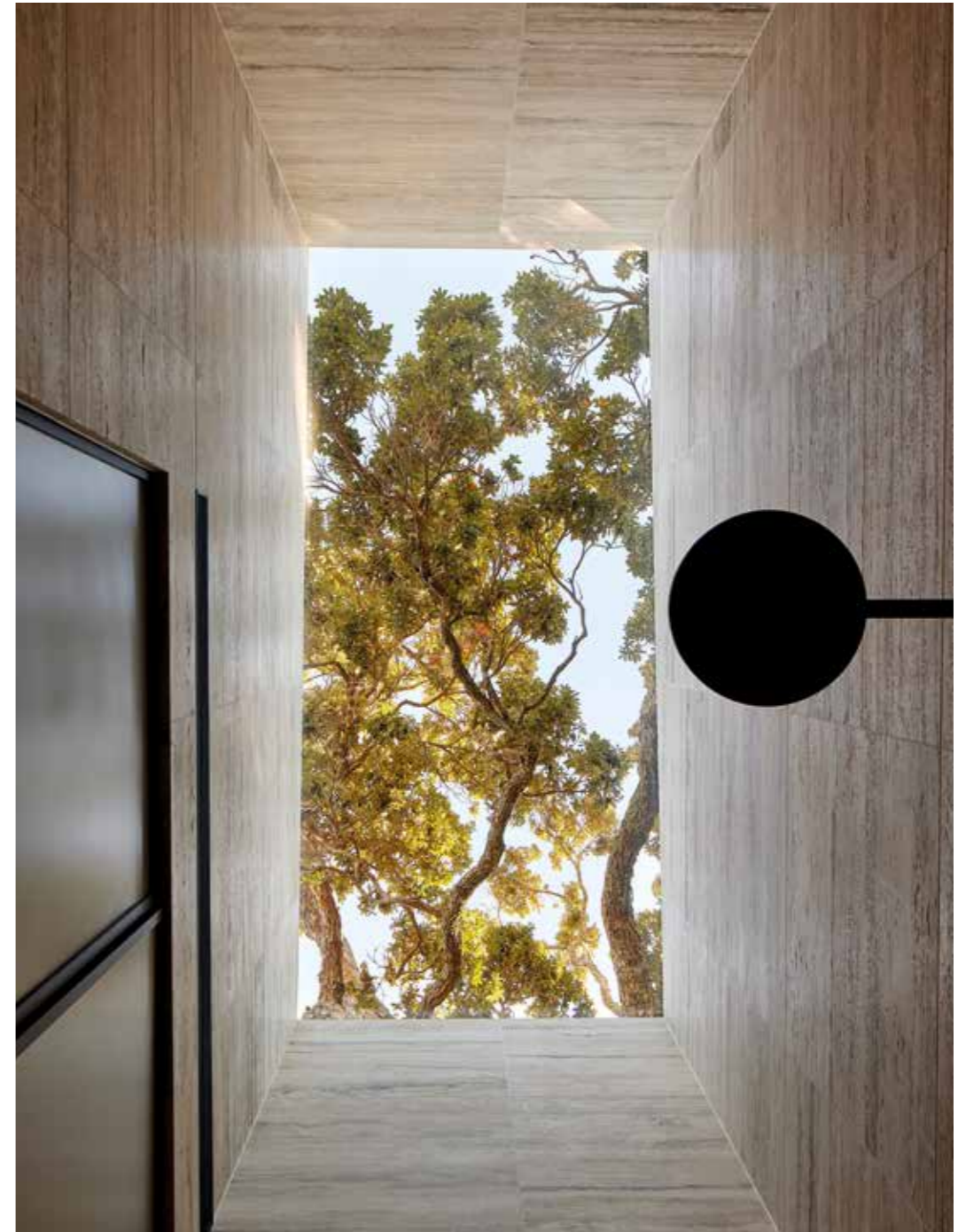
ABOVE Like the one at the entrance to the main living space, this roof window by First Windows & Doors above the ensuite shower is thermally broken to retain heat. Its ThermalHeart technology sees an additional insulator stitched into the core of the aluminium window system, keeping warm and cold areas separated for a drier, healthier home that's cosier in winter yet cooler in summer. OPPOSITE With narrow frames designed to maximise the view, more APL Architectural Series sliding doors and custom windows combine with First Windows & Doors louvres in the main bedroom. This sleep space (and the laundry beside it) has the pleasure of its own private deck, which borrows an elegant view of the neighbours' tennis court without sacrificing privacy and provides an external connection to the home's lower level.
