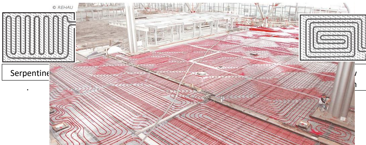
Figure C6.5. Commercial Radiant Floor Heating System (Before installation of upper slab).
